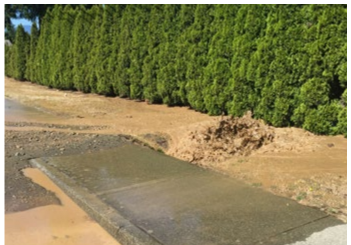
Above: Water main break along Johnston Road
