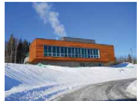
UNBC's BioEnergy Plant uses wood waste from a local sawmill to produce energy for heating the university
