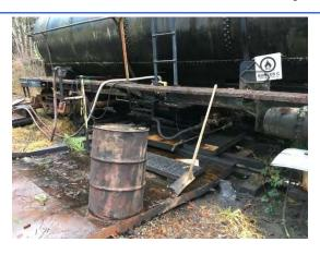
**Photo 9.** Secondary containment of fuel transfer area under Fuel Tanker Car-18 (APEC 19).
