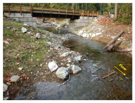
Photo 16. The completed bridge is designed to convey the 200-year flood. Gravel was placed on top of the riprap and the area was vegetated with grass and tree seedlings.
