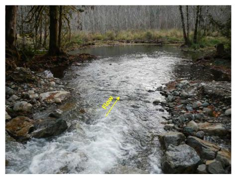
Photo 10. The completed sediment pond dissipates hydraulic energy and helps to settle sediment from the new channel upstream. It provides a good resting pool for fish too.
