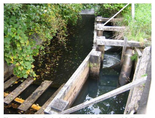
Photo 6. Hatchery Intake (looking down the Fishway and Spillway)
