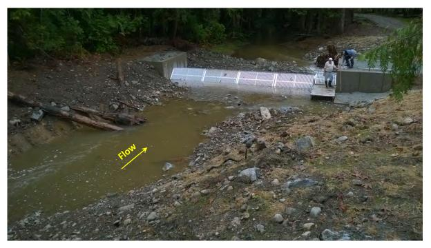
Photo 23. The aluminum fish screens and the old fish trap box were reused.
