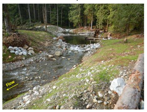
Photo 29. The channel banks were seeded with grass seed to reduce surface erosion, and planted with tree seedlings to help establish a future riparian forest.
