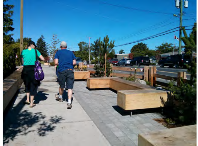
Recently installed mid-block curb extension to create a seating area (within a MOTI right-of-way).
