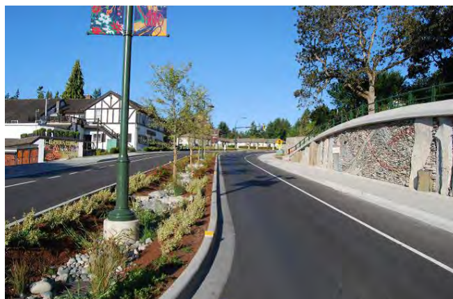
In View Royal, the Island Highway upgrades incorporate stormwater management facilities within a central planted median.
