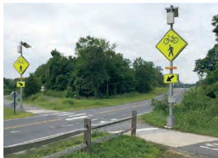
Examples of pedestrian activated, solar powered crossing signs with flashing lights for visibility. (image credit: Eltec Corp Traffic Products)
