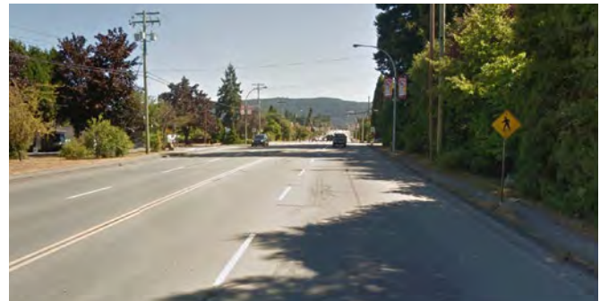
Existing conditions with extra wide curb lanes, galvanized cobra lighting with banners, overhead utilities, and no sidewalk on south side (see Recommendation 5).
