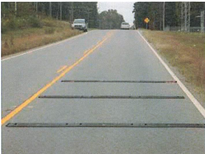
Example of Temporary Transverse Rumble Strips
