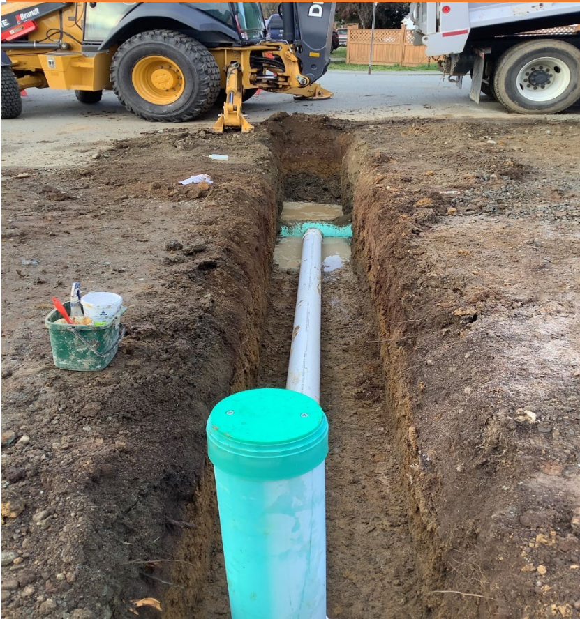
Figure 1: New Storm Connection Installation on David Street
