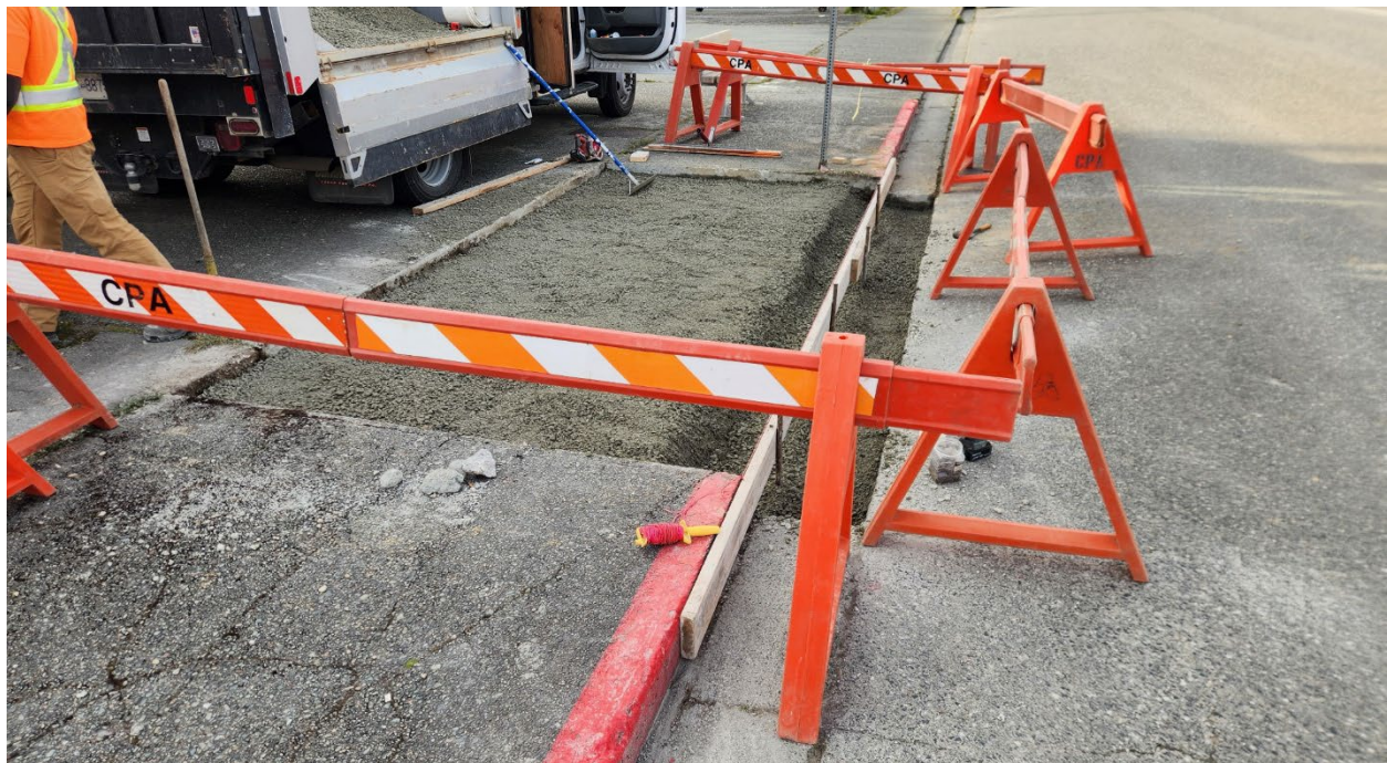
Figure 2: Sidewalk Construction for Upgraded BC Transit Shelter
