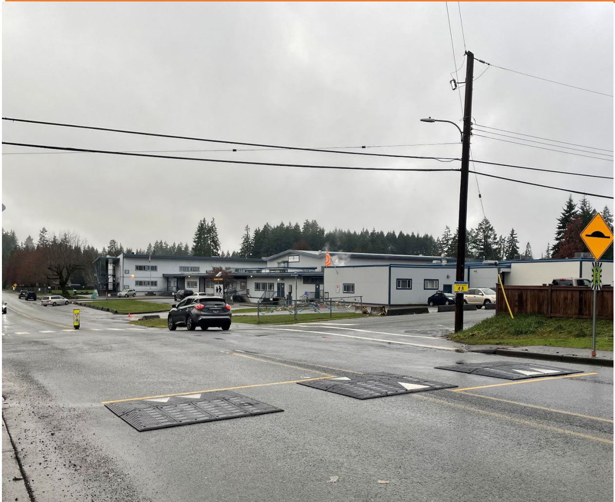
Figure 3: New Speed Humps on Compton Road in Front of Tsuma-as Elementary School
