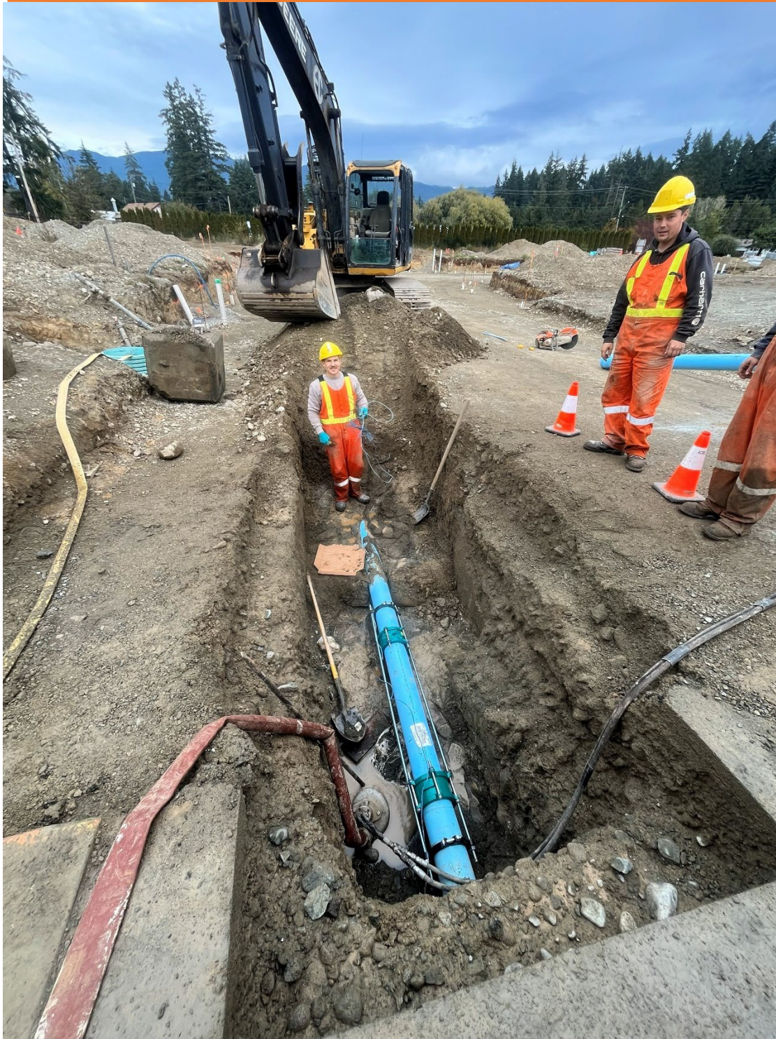
Fig 1: New 150mm Water Tie-in for Pierce Road Subdivision
